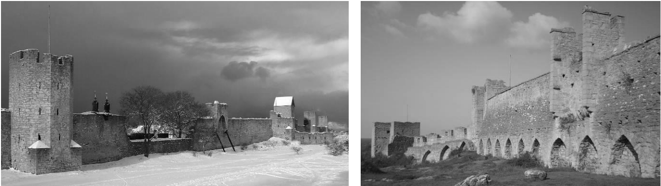
Figure 1. Visby City Wall seen from outside and inside. The smaller wall towers are riding on top of the wall. In many places one can see old collapses as well as different kinds of reinforcing structures.
