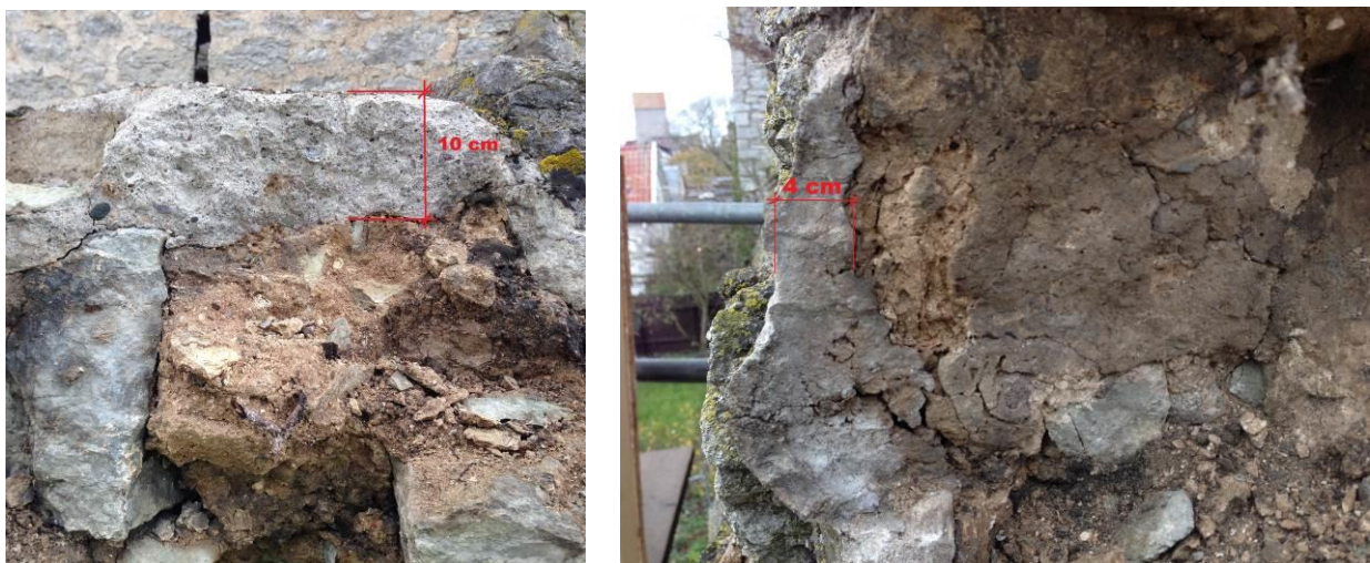
Figure 5. The first picture is showing the concrete cover on top of the wall, and directly beneath it is the type (c) mortar. Here this mortar was more deteriorated and more wet in approx. half a meter from the concrete layer than it was in general – not surprising for a 700 year old lime mortar situated on top of a wall. The second picture is showing the cement mortar covering the old lime mortar, showing the area of lime mortar just behind the cement as deteriorated in a thickness of approx. 5 cm.
