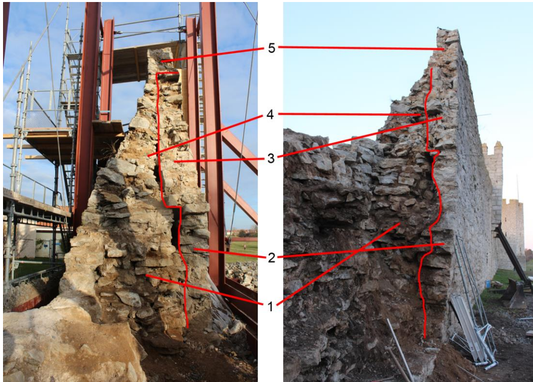
Figure 3. Two photos showing the same part of the wall at two different stages during dismantling of the collapsed part. 1) Lower core with clay mortar and no bond. 2) Thin outer masonry leaf. 3) Former parapet now outer leaf of middle part of the wall. 4) Upper core inside parapet wall. 5) Top with solid masonry.
