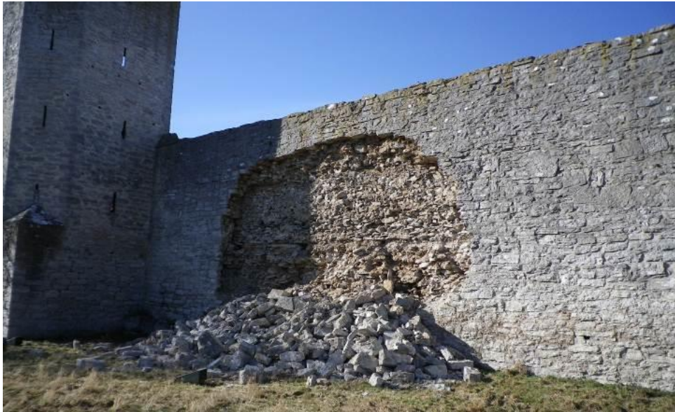
Figure 8. Visby City Wall in 26th of February 2012, a couple of days after the collapse.
