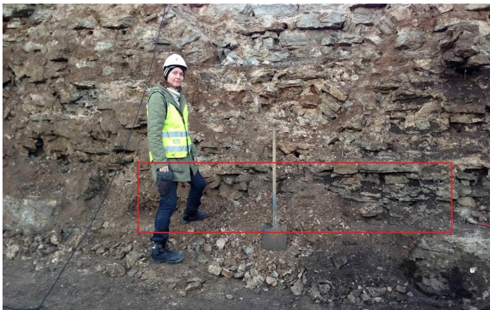
Figure 9. The area where the collapse probably started is a part of the wall where the masonry leaf was no thicker than a foot length, see the marked area. No binding stones were used in this part.
