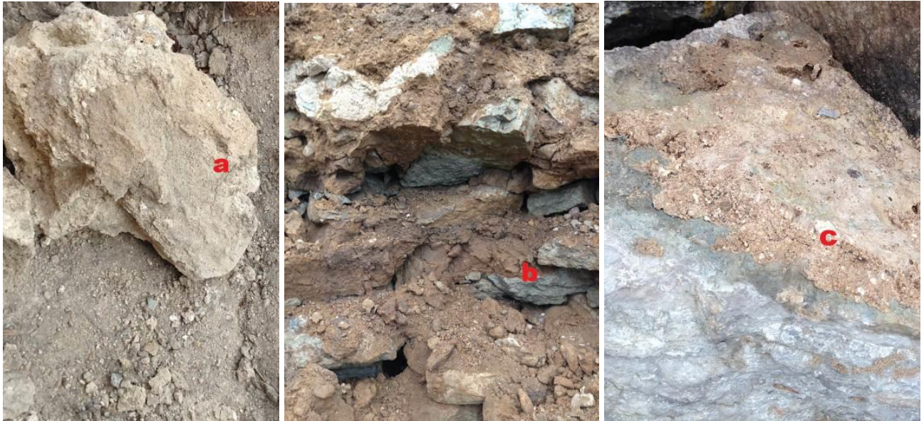
Figure 4. The fat lime mortar (a) is white and rather homogeneous. Lots of smaller lime lumps exist. It has a good adhesion to the limestone. The clay mortar (b) of the wall core is in good condition, powdering when dry and stable when wet. It has filled up the stone core very well. The type of mortar used in the second building phase (c) has a very good adhesion to the lime stone and is in general extremely well preserved despite its exposed position.
