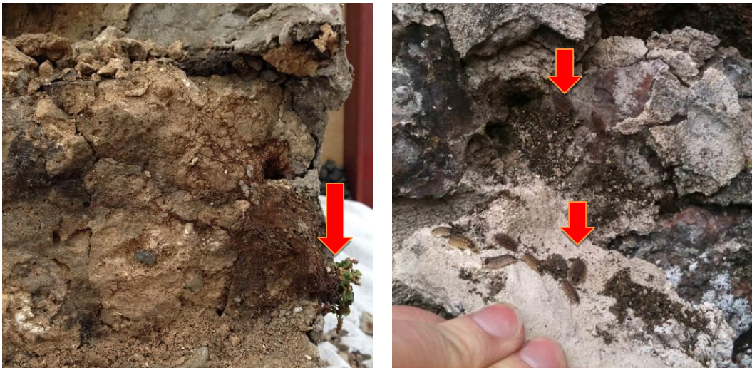
Figure 7. a) A small plant with a large root system reaching far inside the city wall. It has been able to grow first after the joints were repointed with cement mortar. b) Woodlice found in the moist environment behind cement mortar.
