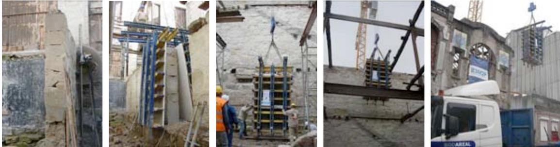
Figure 7 : Panels for laboratory tests (from left to right): cutting, extraction and transportation
