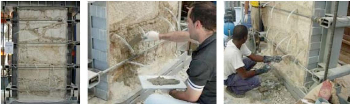
Figure 11 : Injection of the mortar in the panel PP3.
